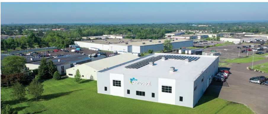
The Aeroseal facility in Miamisburg, Ohio
