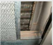
Figure 3: Metallic filter with one-inch thickness and two-inch gap
