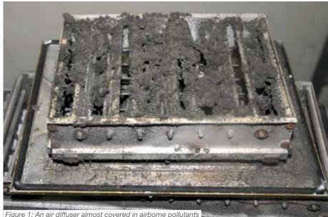
Figure 1: An air diffuser almost covered in airborne pollutants
