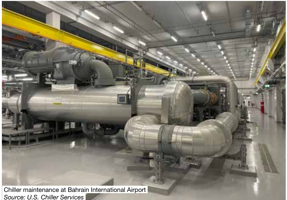
An Operation & Maintenance engineer at work Source: Dalkia Middle East
